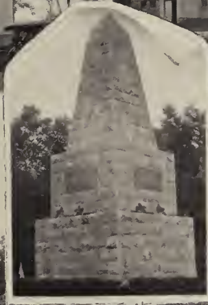
EASTERN BRANCH NATIONAL HOME D/S
